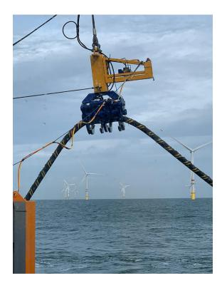
**Rotech Subsea** were contracted by **Van Oord** to provide the Hydraulic Powered RSG1 Cable Grab tool for the recovery of multiple Fibre Optic and Inter Array cables to the vessel deck. Operations were carried out at Norther Offshore Windfarm.
